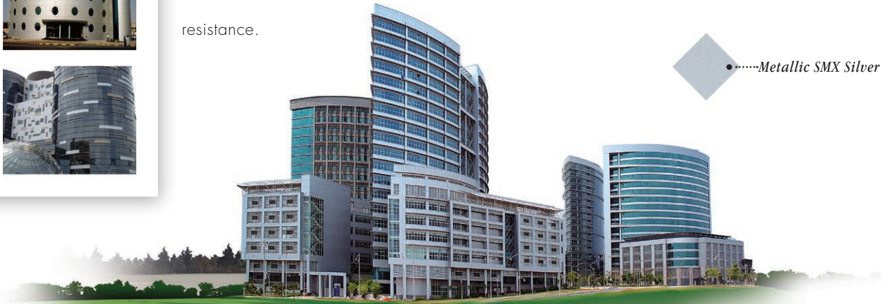
FEDERAL GOVERNMENT ADMINISTRATIVE CENTER PUTRA JAYA, MALAYSIA
